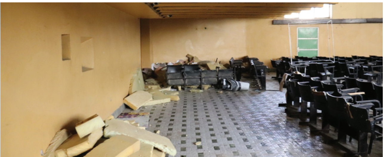
Some other scattered archival materials at the corner of the meeting hall. The meeting hall is in active use for several purposes.
